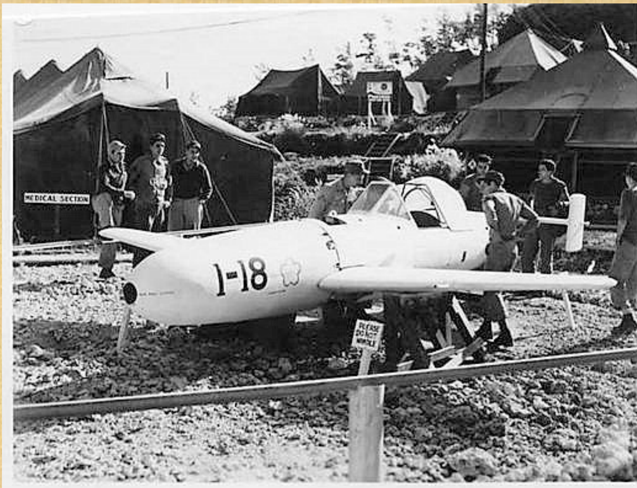
112th SEABEES WEBSITE PHOTO PINETREE ARMY AIR BASE SIGN IN THE BACKGROUND AS IN PHOTO ON PAGE 1
